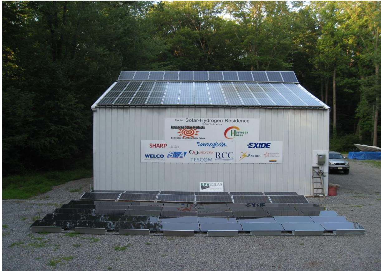
14 kW PV panel array
